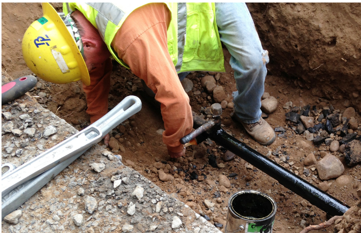
UTC pipeline safety inspector.
